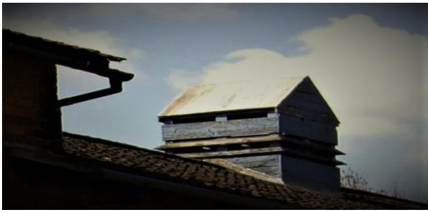
Photo of bell tower the Old School House, Lambley
