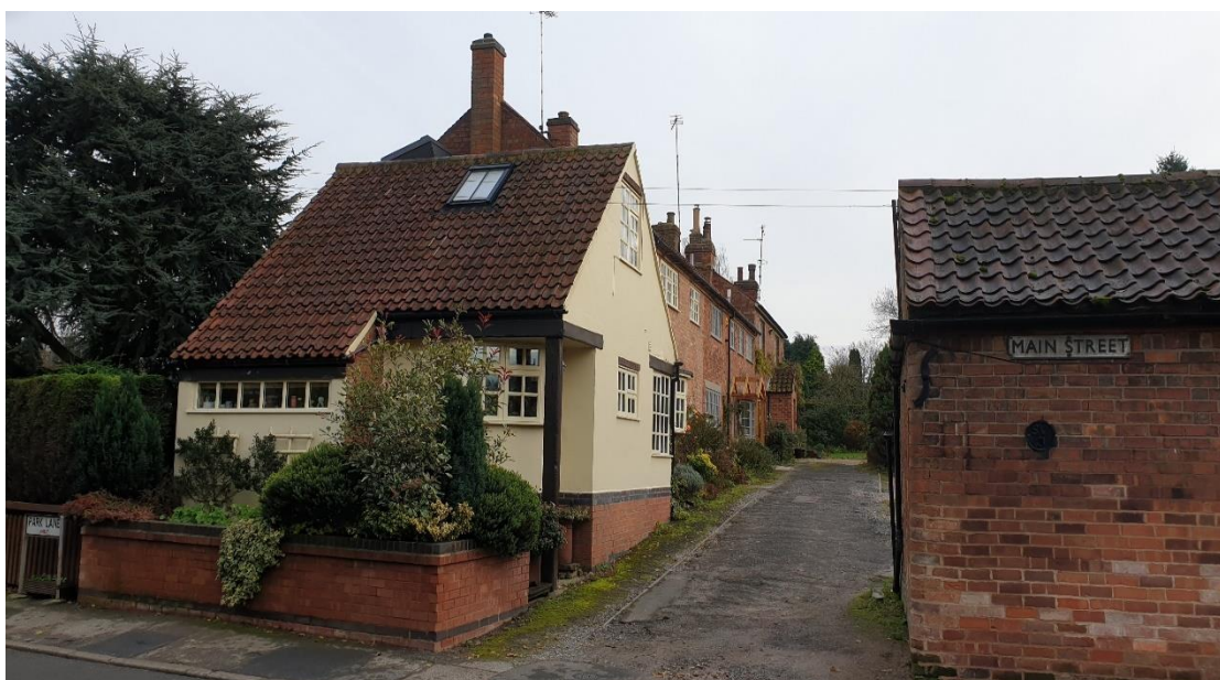
Photo 37: Nos 1 to 3 Park Lane
