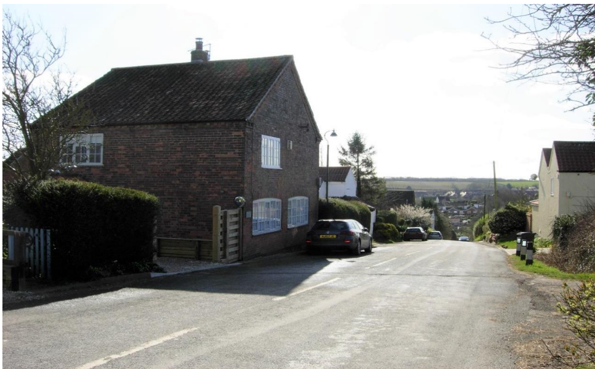
Photo 49: View south down Green Lane with 38 Green Lane left number 38 with the double gable is on the right and number 30 the white rendered cottage in the background.
