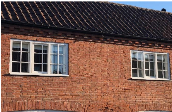
Photo of 18 Main Street with horizontal Yorkshire sliding sash windows.
