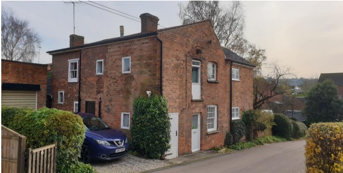
Photo 29: No 45 Main Street
