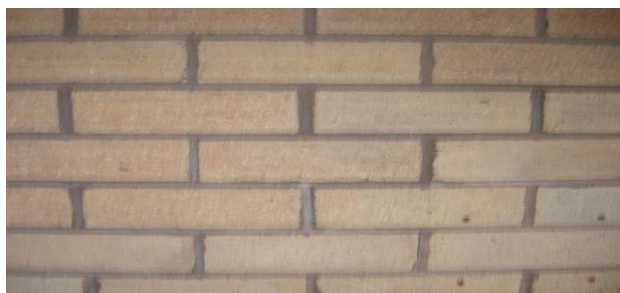
Photo of stretcher bond type brickwork
