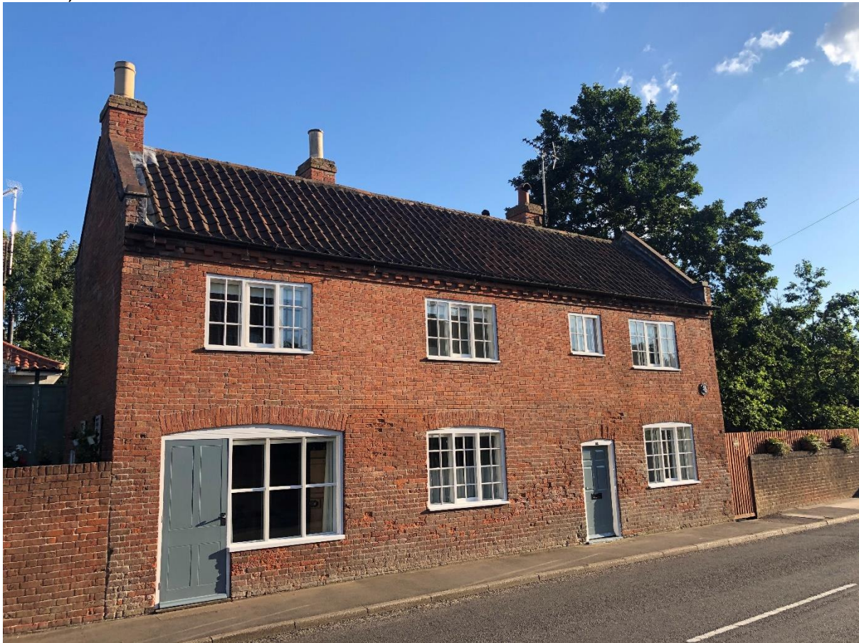
Photo 28: No 18 Main Street
