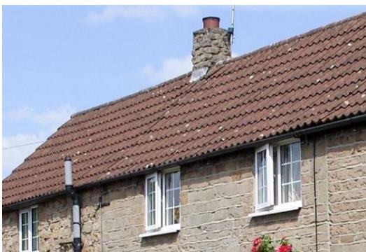
Photo – casement windows
