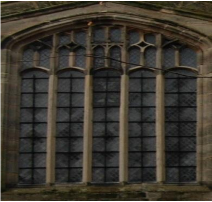
Photo Tracery window on east façade of Holy Trinity Church
