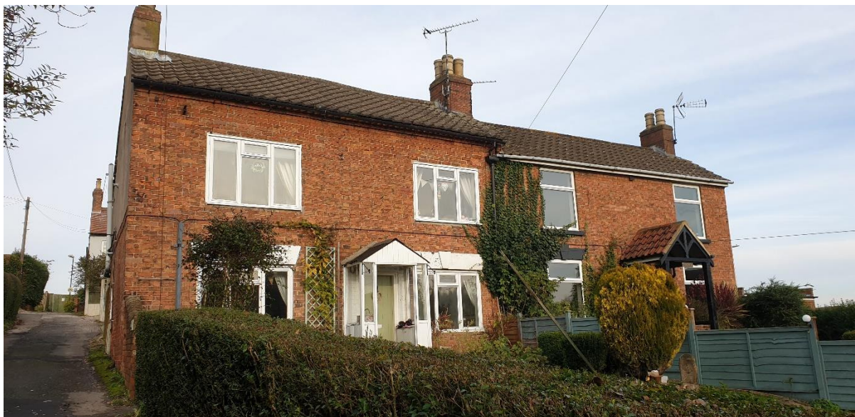
Photo 53: Cottages on Chapel Lane
