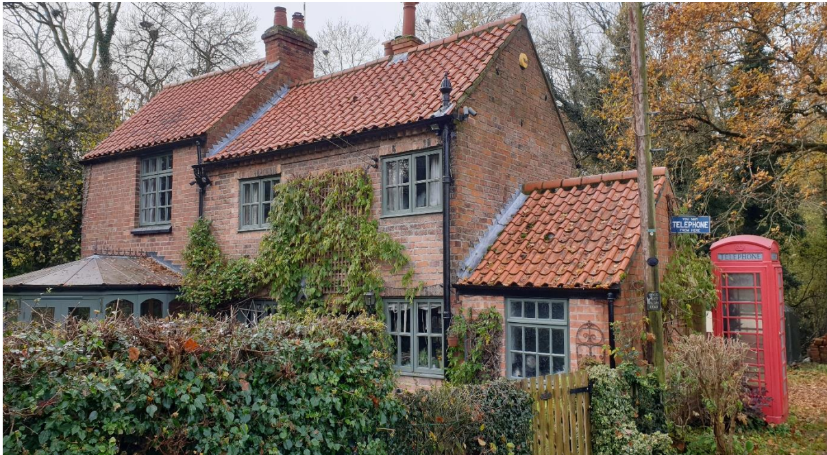
Photo 56: Dumbles Cottage at the west of the Conservation Area - note K6 phone box but probably not in original location
